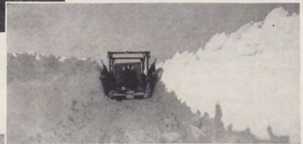
Crews worked in tough Maine weather to complete the conversion job by spring. In 26° below zero weather a town plow opens up the road for telephone crews.
