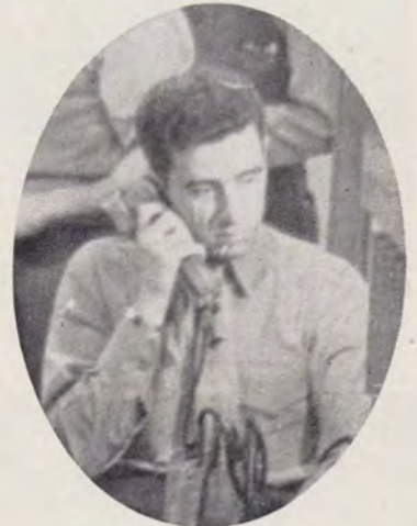
Ray Heyliger, shown at the frame, tests the wiring just before the cutover is made official.
