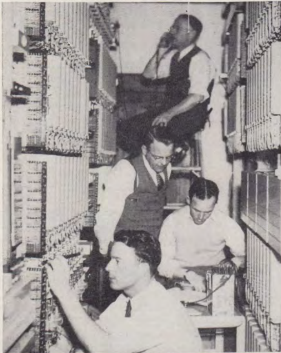
Working on the frame in the new Livermore Falls Office are, from top to bottom of picture: Charles Daniels, Nat Chase, Equipment Foreman; Donald Keating and Ernest Dobson.
